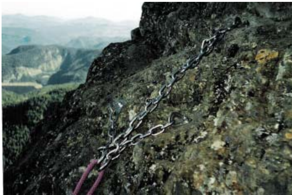
New anchors on the upper belay station
